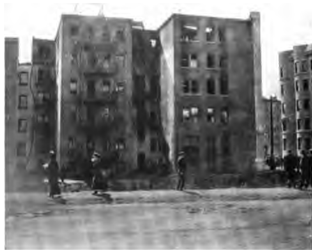
Fig. 2. Apartment House after Fatal Fire.
